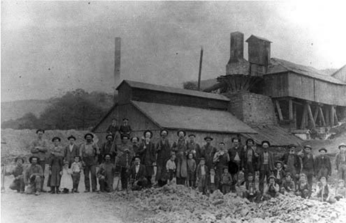
Figure 15. In this historic black-and-white photograph, a large group of men stand in front of a blasted industrial landscape dominated by a huge furnace and buildings at Greenwood Furnace State Park, Pa. ( www.dcnr.state.pa.us/stateparks/findapark/greenwoodfurnace/ ).
